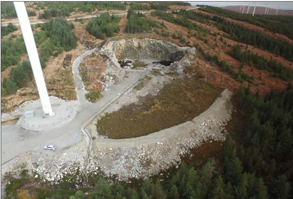
Plate 1: Borrow Pit prior to backfilling (c.2016).
